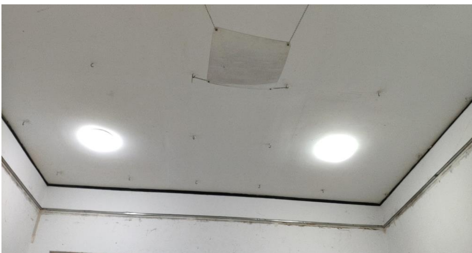
6" concrete slab with no drop ceiling
