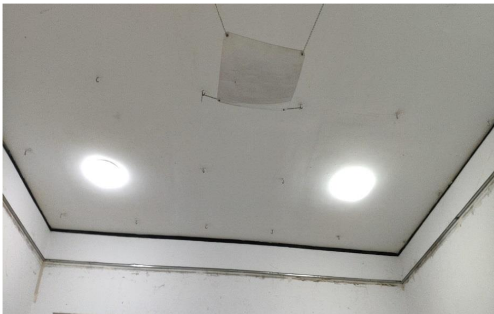
6" concrete slab with no drop ceiling
