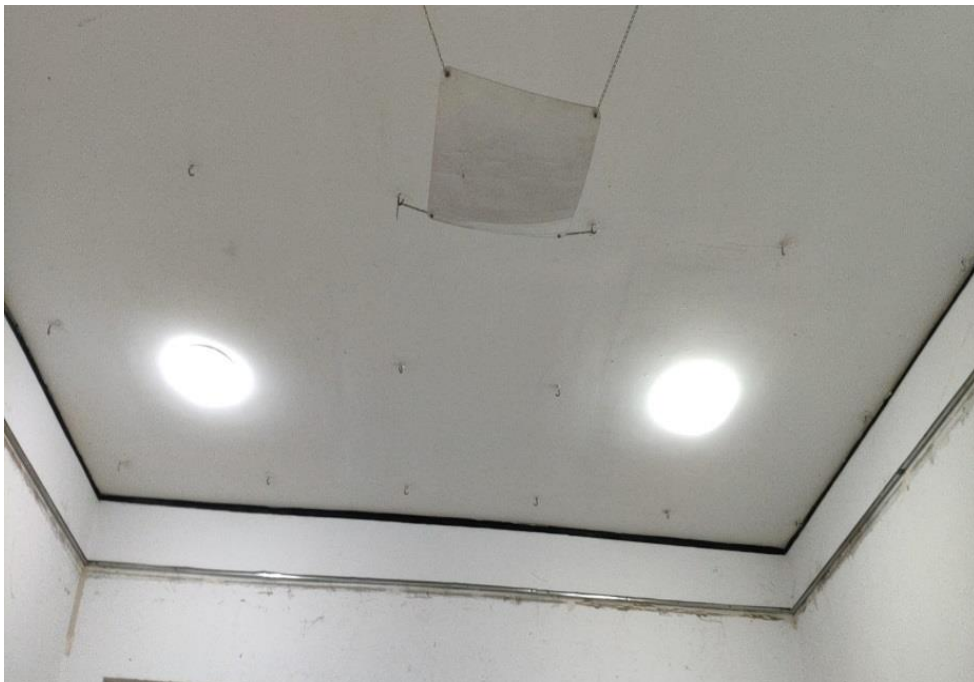
6" concrete slab with no drop ceiling
