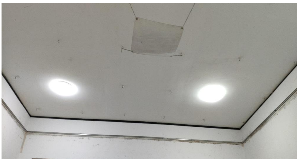
6" concrete slab with no drop ceiling
